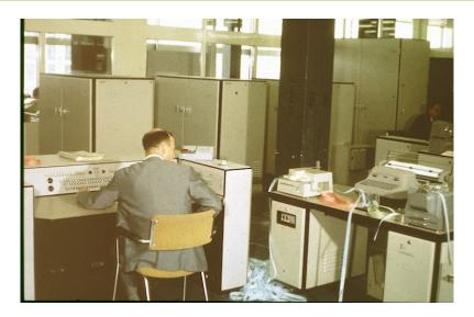
Transistorized, core memory, interrupt, and I/O: Reliable and fast
